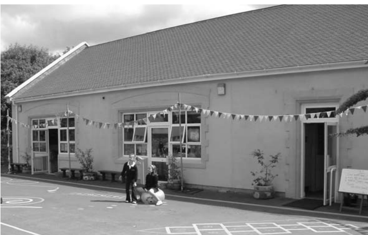
New school extension, 2007
